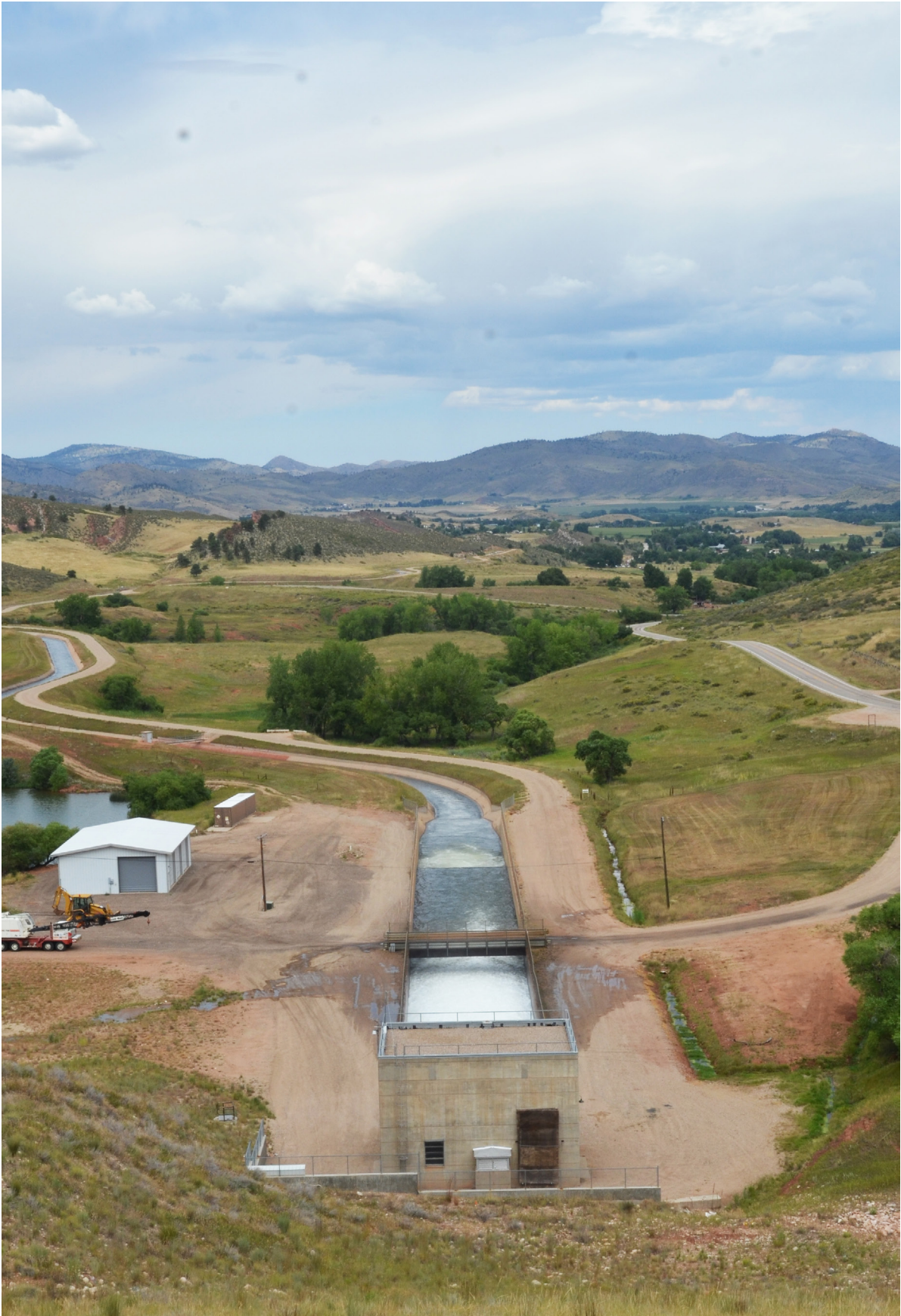
Hansen Supply Canal delivers water from Horsetooth Reservoir into the Poudre River.
