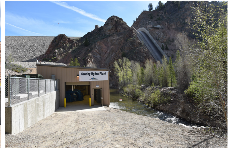
Granby Hydropower Plant below Lake Granby in Grand County
