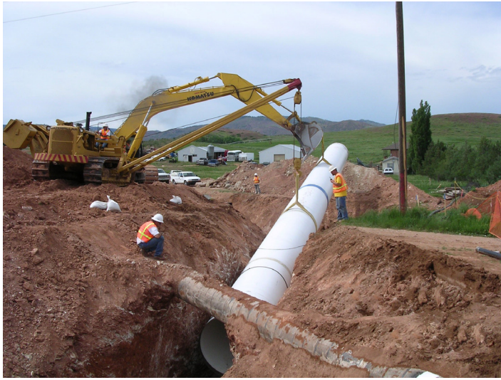
Construction of Pleasant Valley Pipeline
