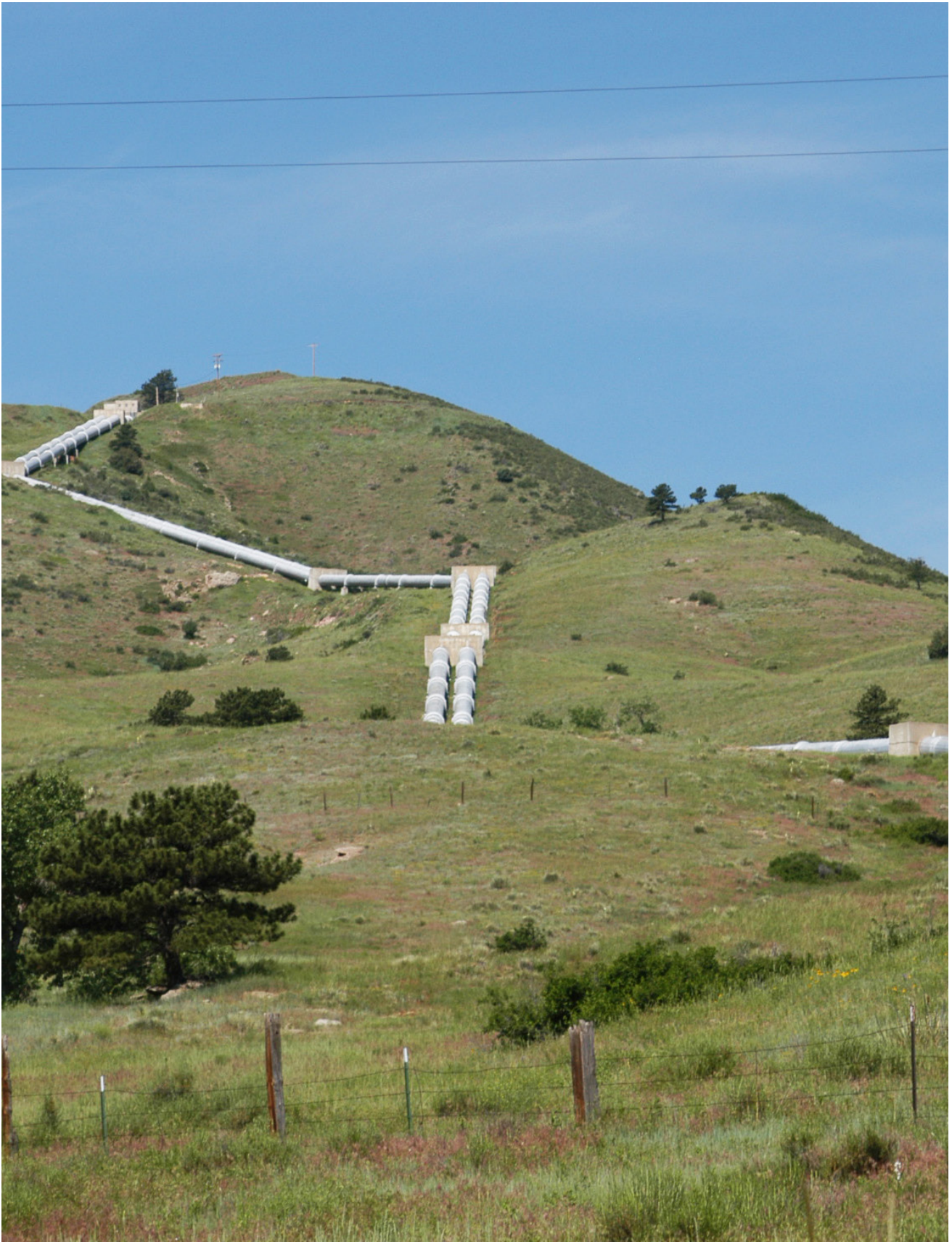
Flatiron Penstocks deliver water from Pinewood Reservoir into Flatiron Reservoir.
