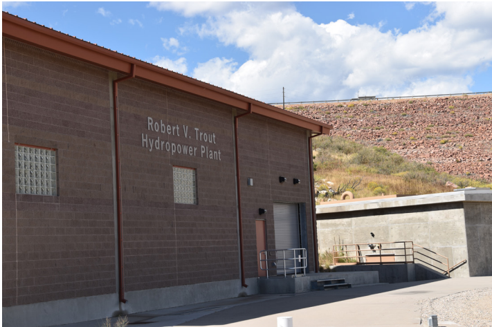
Robert V. Trout Hydropower Plant below Carter Lake in Larimer County
